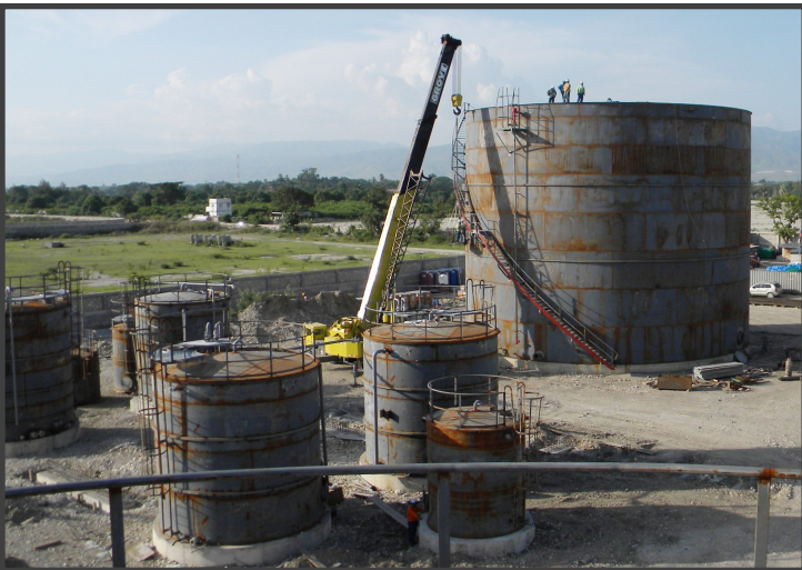
Construction of Tank Farm, Haiti
