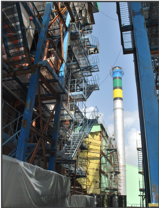
Construction of Gas Cleaning Equipment, C.A.
